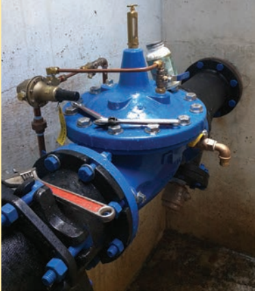
Pressure Reducing Valve being installed
