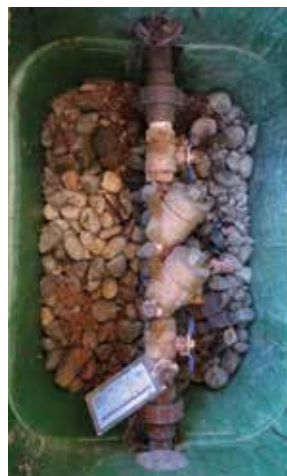
Backflow Assembly being tested
