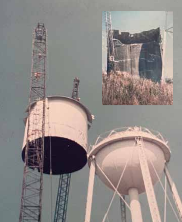
Removal of our old 50 thousand gallon reservoir and the adjacent 1 million gallon reservoir in preparation for a new 3.7 MG reservoir and Booster Pump Station.
