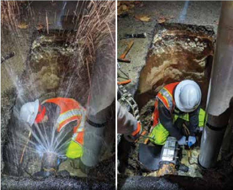
Before and after the repair of a water main after soils shifted underground.
