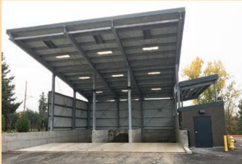
A separate Decant Facility allows our vactor truck to empty its tank on a sloped concrete pad, where the debris can be washed, separated, and dried before being removed.
