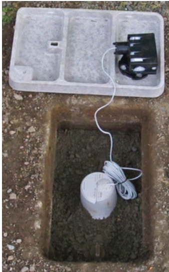
New electromagnetic meter, part of our automated meter reading system
